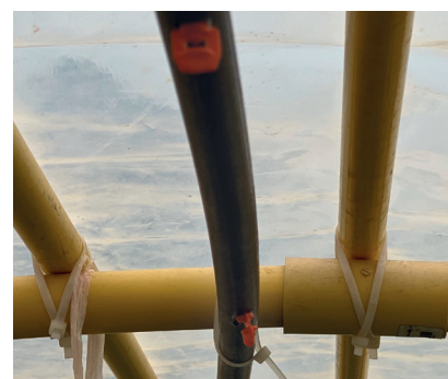
Irrigation pipe Irrigation pipe (9m X 3) with mister or microsprinklers ( X 50)
